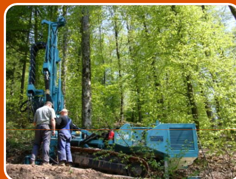
Germany - Core Drilling \phi 101.6\text{mm} Deutschland - Kernbohren \phi 101.6\text{mm}
