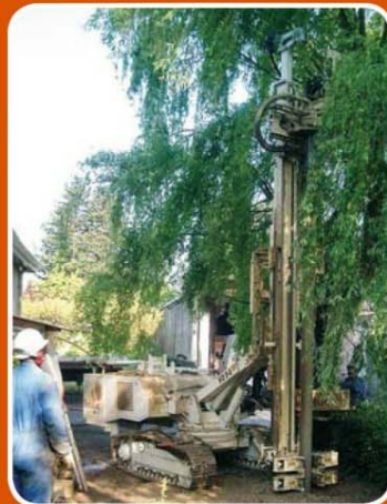
Malaysia - Down the Hole (DTH) Hammer Drilling \phi 273.0\text{mm} Malaysia - Im-Loch-Hammerbohren \phi 273\text{mm}
