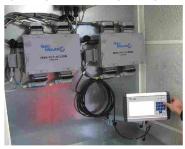
**IPER-PVP-VISION** is a system for the measuring, storage and control in the soil consolidation process with concrete injections; the system can control up to a max of 8 injectors.
