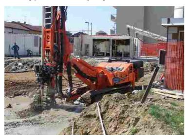
The central unit includes a push-button to disable depth measuring when the change of the drill rod is required. This changes of the rod can also be performed automatically using a pressure switch.
